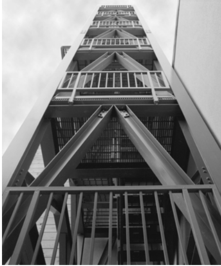
Figure 7-3. Pultruded composites frame structure. Source: Courtesy of Strongwell Company, USA.
