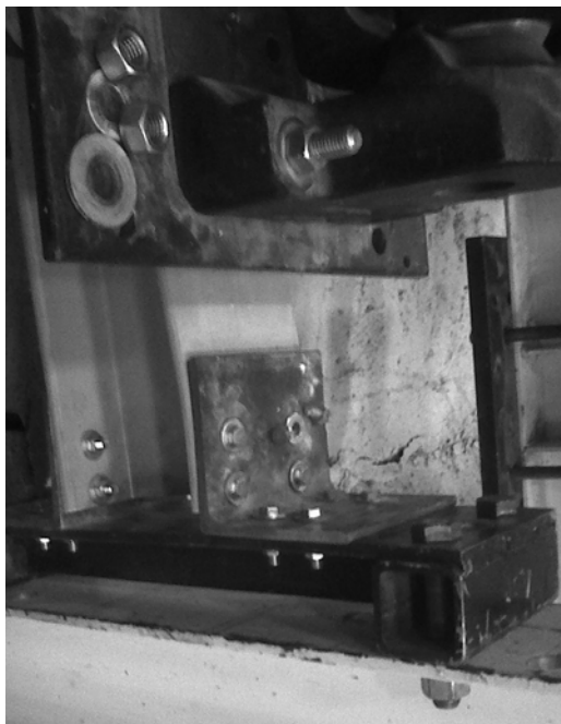
Figure 7-131. Failure of connection 2. Source: Mosallam et al. (2010a).
