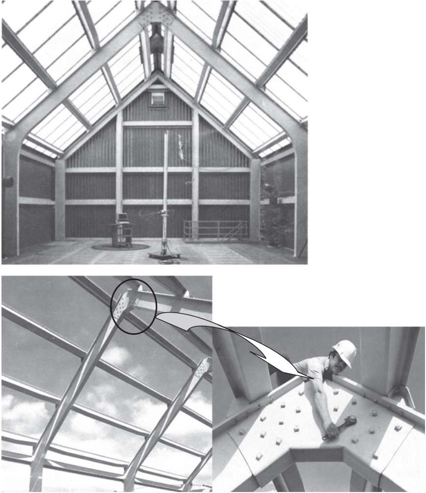
Figure 7-7. A portal frame fabricated according to Enduro Tuff Span connection details.
