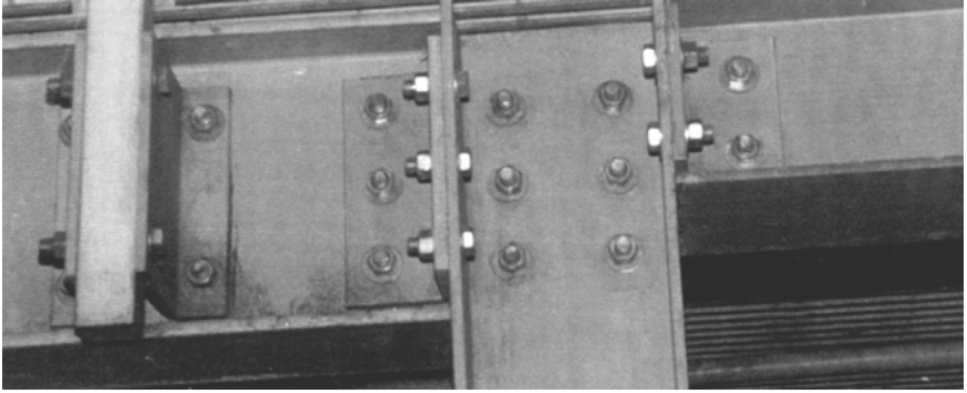
Figure 7-5. An example of “steel-like” frame connections.
