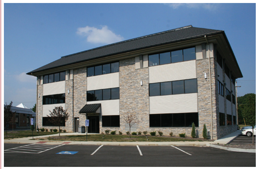
Figure 23 A three-story masonry bearing wall building.
