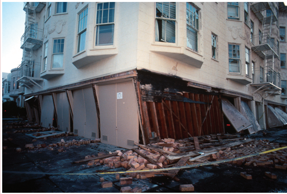
Figure 18 First story of an apartment building in San Francisco, California, leaning to the side after the 1989 Loma Prieta earthquake.
