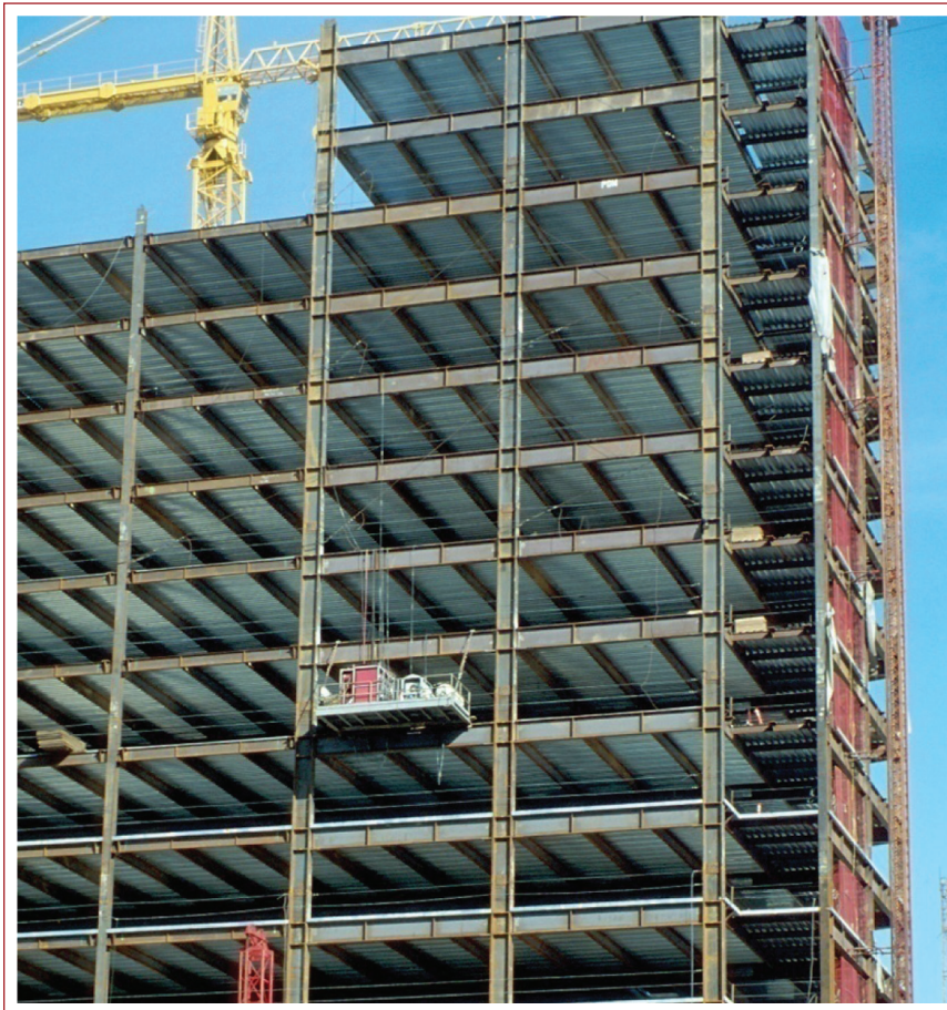
Figure 25 A tall steel moment-frame structure under construction.
