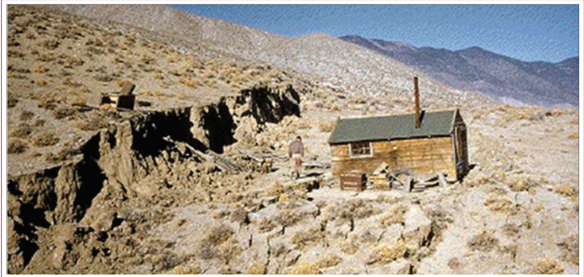
Figure 4 Vertical fault offset in Nevada resulting from the 1954 Dixie Valley earthquake (photo by K. V. Steinbrugge).
