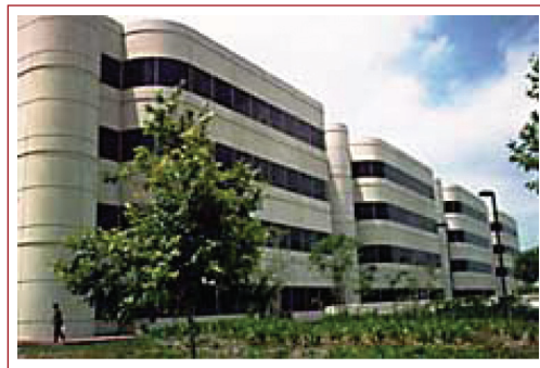
Figure 28 The San Bernardino County Justice Center in California was one of the first base-isolated buildings in the United States.
